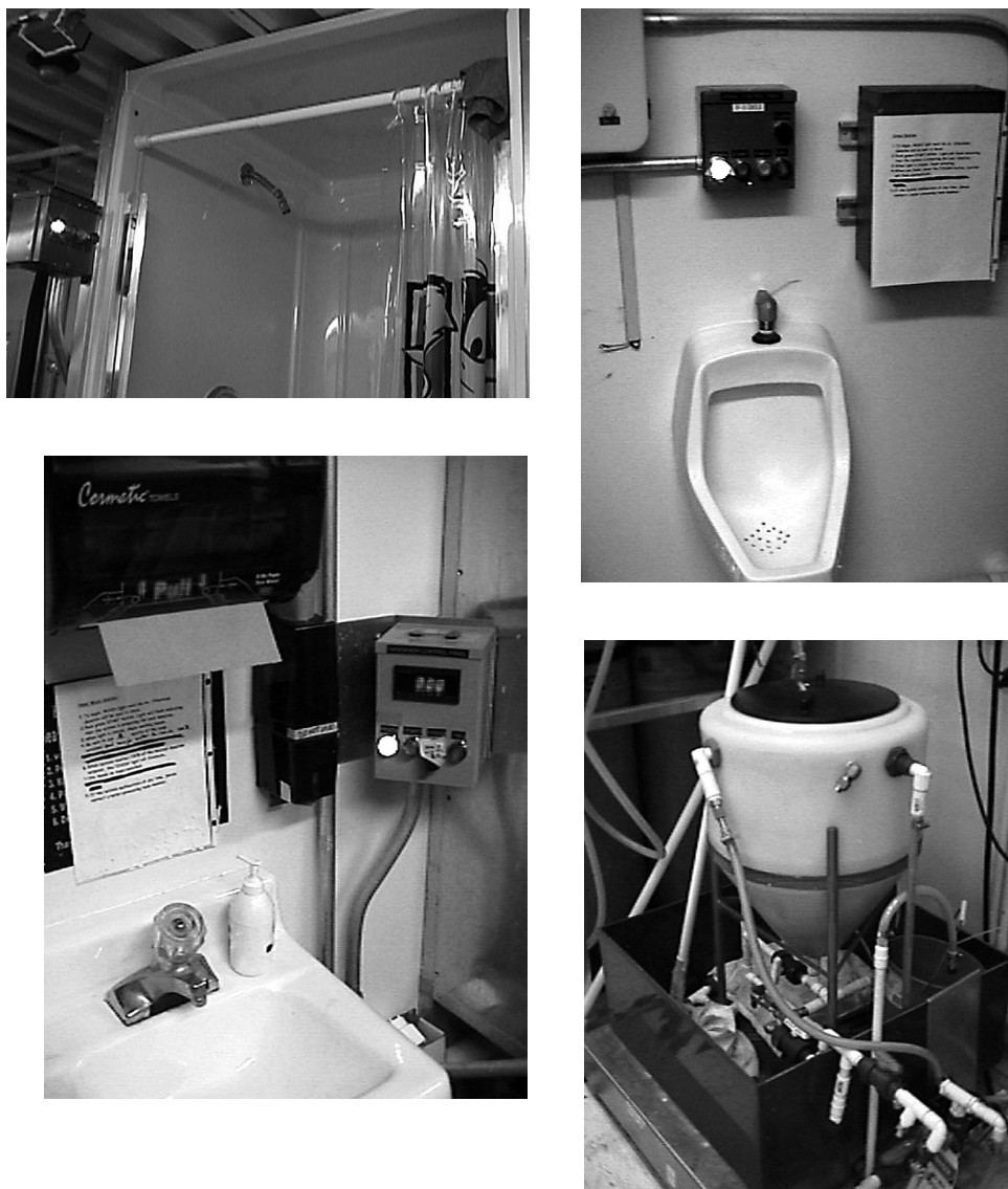
Figure 3. The Integrated Water-Recovery System Waste-Water Collection System.
